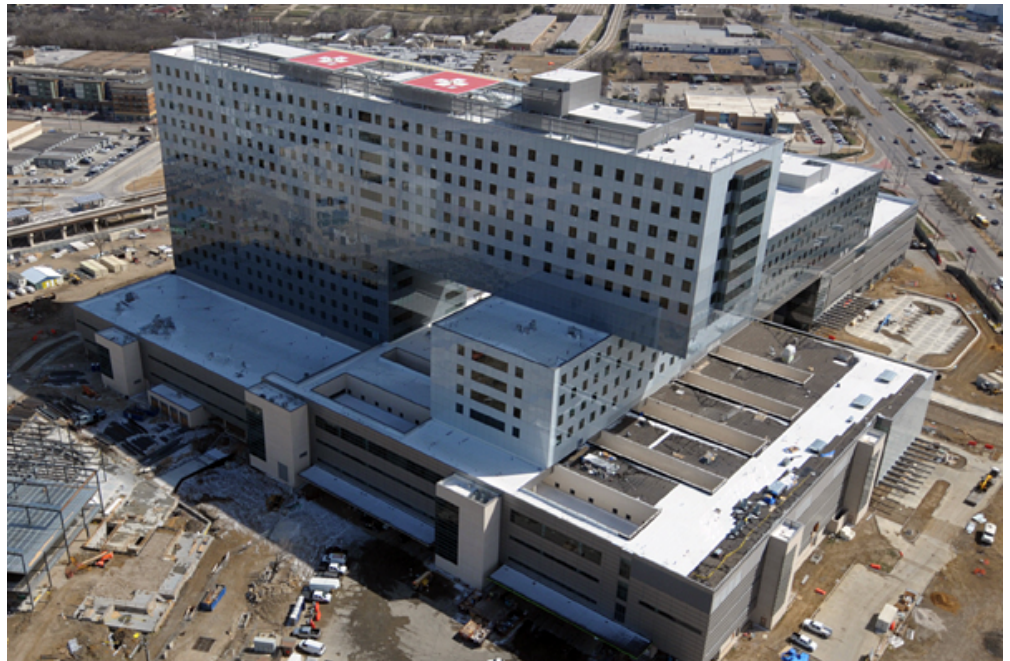
Parkland Hospital under construction
