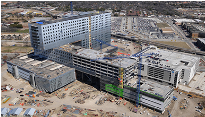
Parkland Hospital under construction
